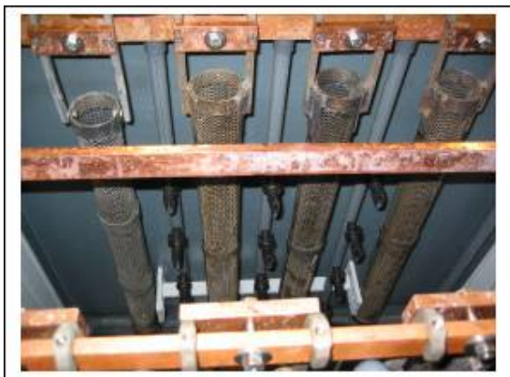
Figure 11: Eductors installed with flow directly towards the cathode.
