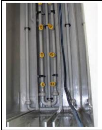
Figure 10: Installation of Eductors in vertical Inpulse line.
