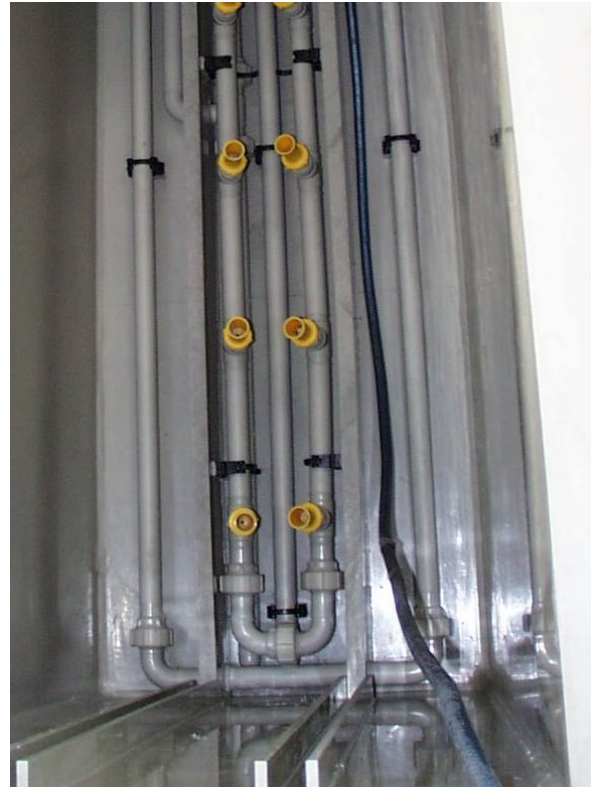
Figure 5: Installation of Eductors in a plating cell
